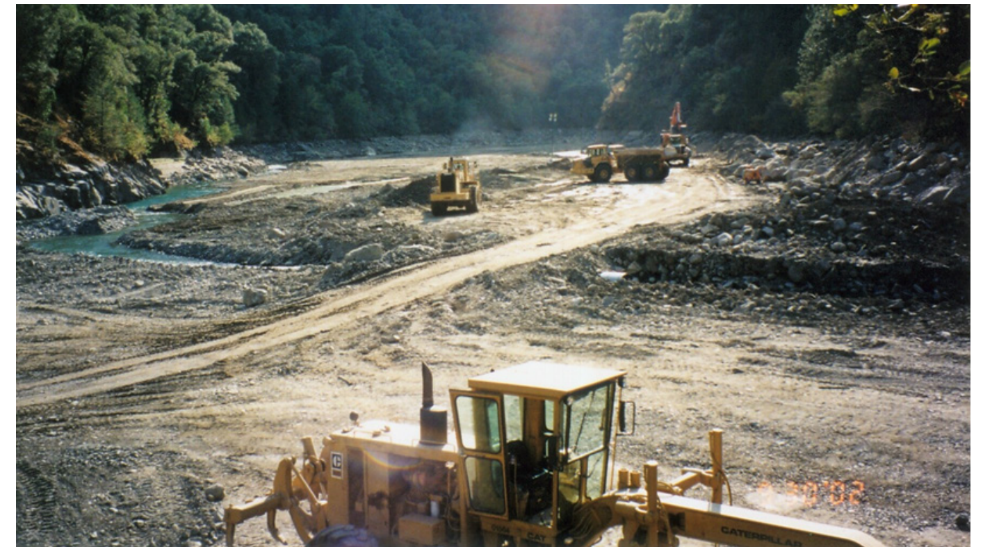
Sediment removal operation at PCWA's Ralston Afterbay facility. © PCWA
