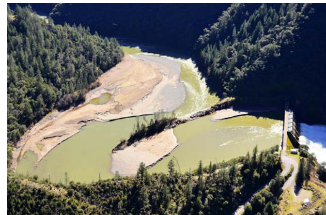
Sediment and debris build up near PCWA Ralston AfterBay Dam. © Placer County Water Agency
